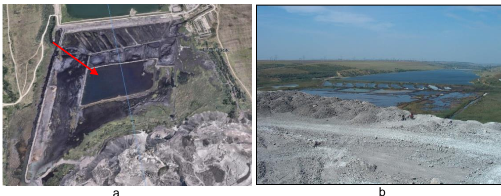
Fig. 4 Lake Mălina North with the location of the wastewater treatment ponds: a - general view (image Google earth, 2021); b - general view, year 2008 (Bălan, 2010).
